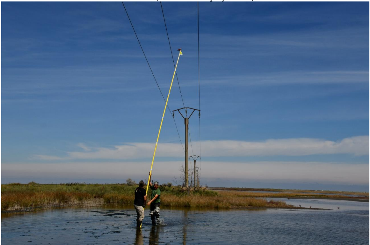
Installation of bird diverters in Romania (ROSPA0031 project site):
