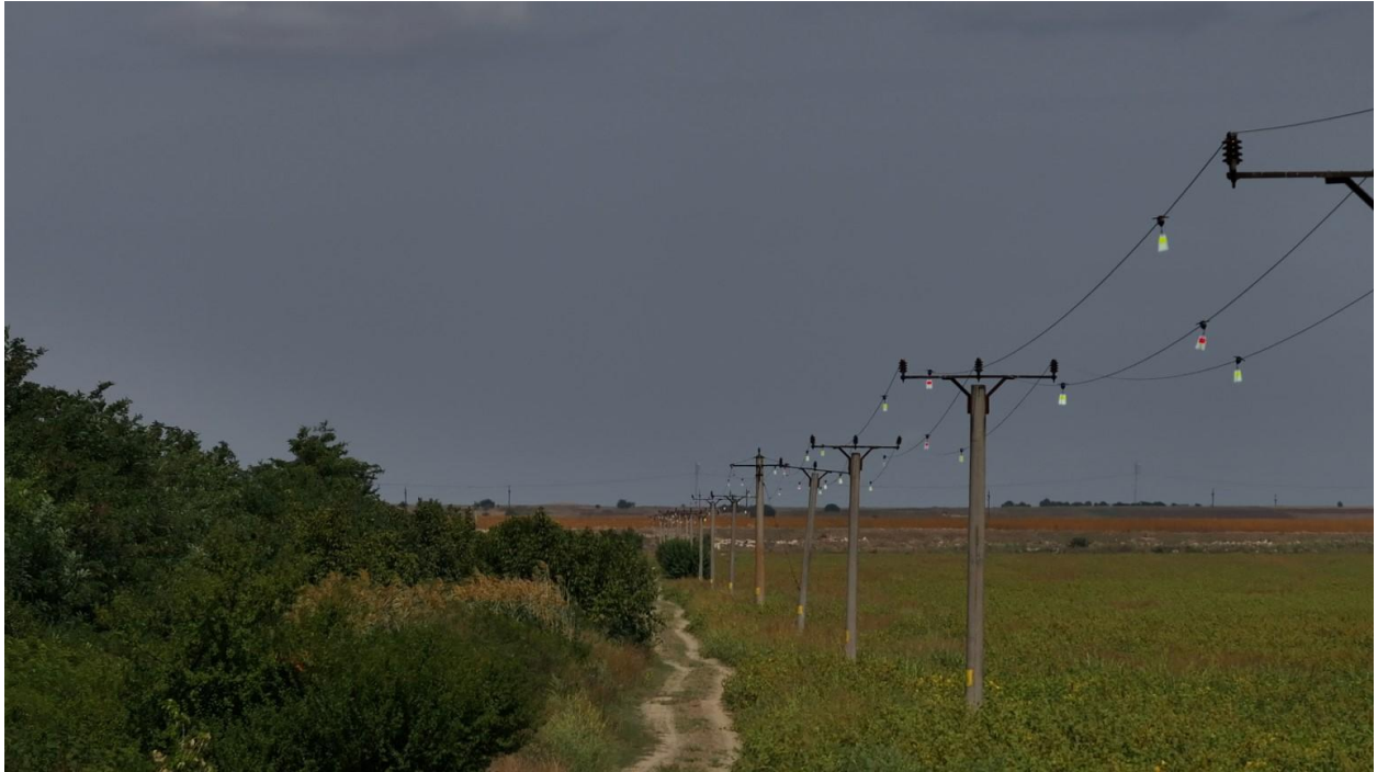
Installation of bird diverters in Romania (ROSPA0031 project site):
