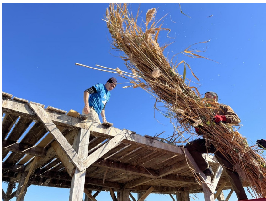
Figure 20. Covering the platforms with reed, Peschina Marsh, 2024.
